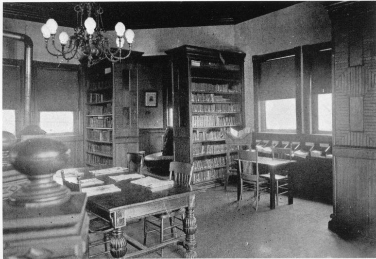
NORTHEAST CORNER (HISTORIC IMAGE)
