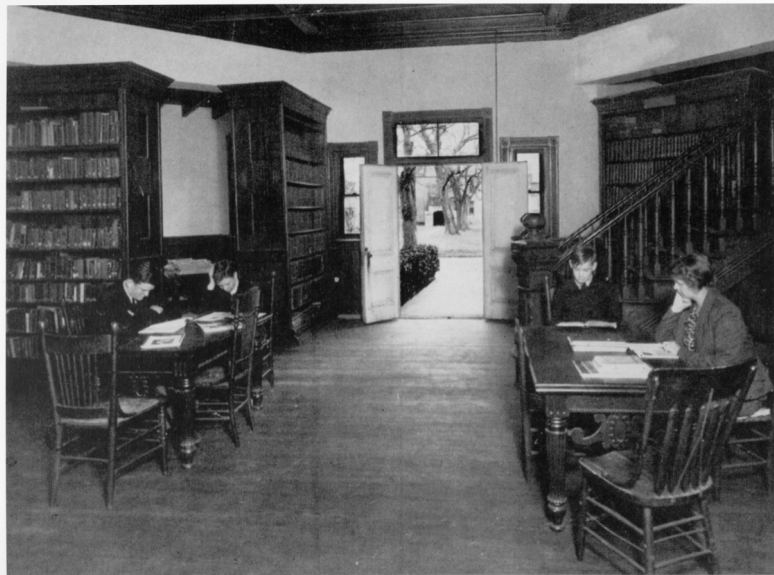
SOUTH WALL INTERIOR (HISTORIC IMAGE)
